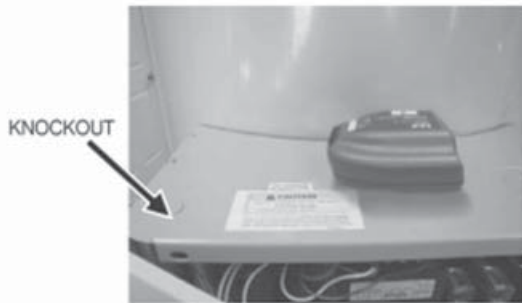
Figure 20. Location of Communications Wiring Knockout
